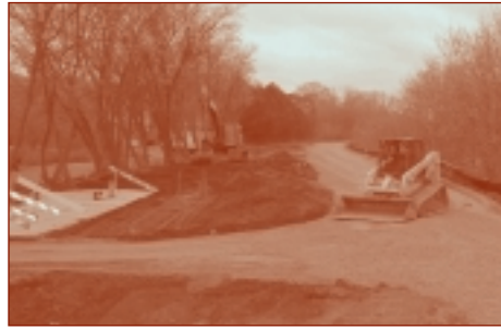
Construction is currently underway on the trail connection.
